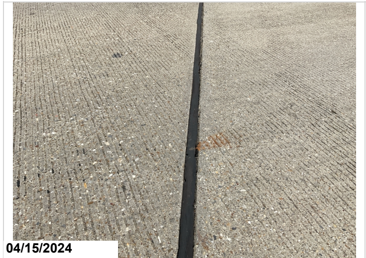
Bent 2, Left side, Loss of seal adhesion, CS2
