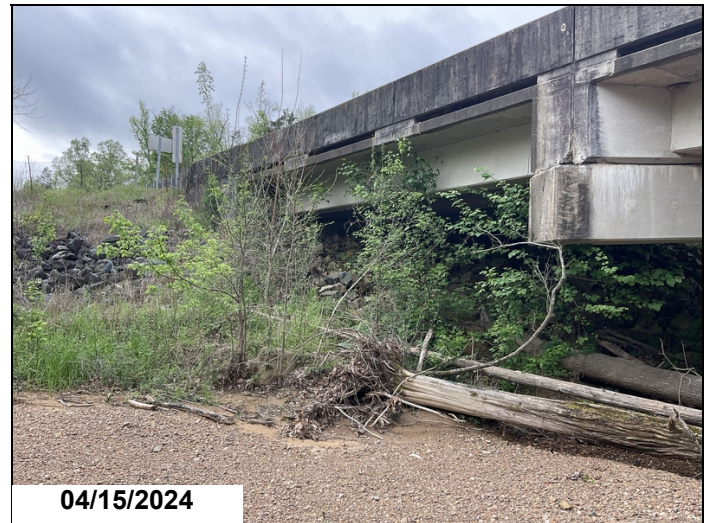
End of bridge, Left side, Trees and vegetation growing over bridge railing.
