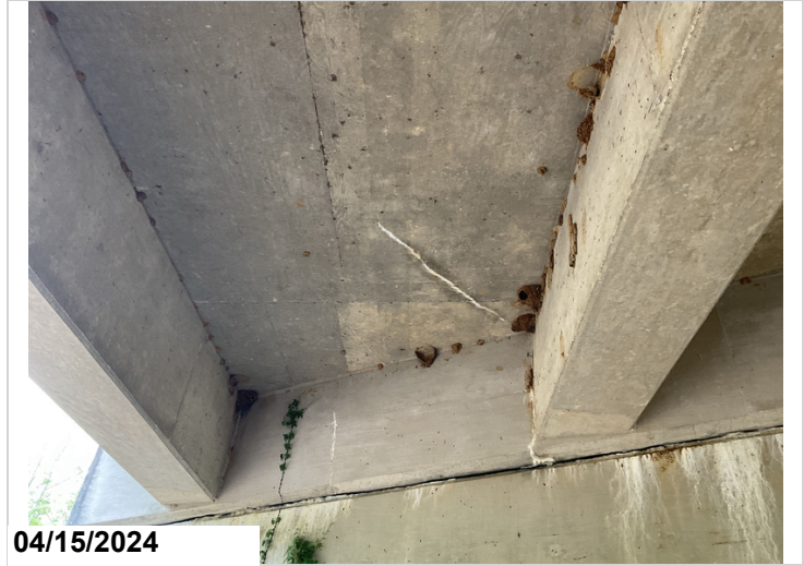
Span 3, Bay 1, cracking with efflorescence to undersurface, CS2.
