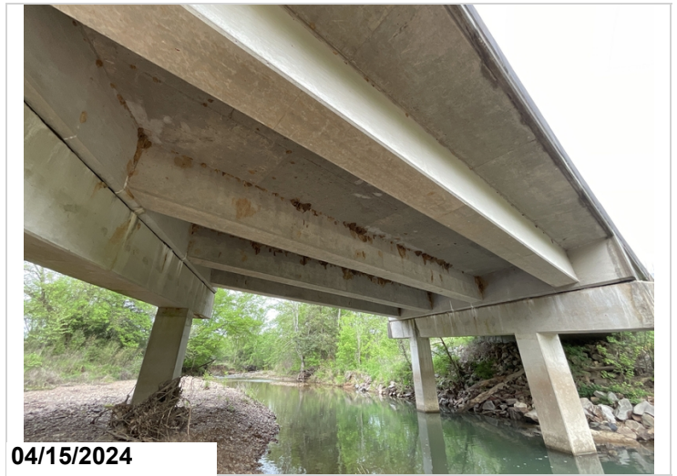
Typical concrete tee beam photo
