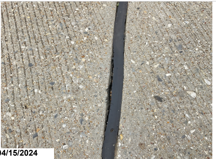
Bent 2, Left side, Loss of seal adhesion, CS3
