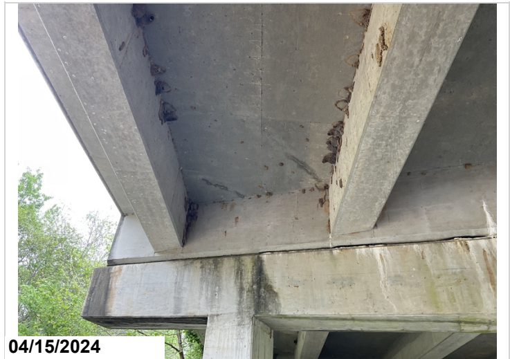
Span 2, Bay 3, cracking with efflorescence to undersurface, CS2.
