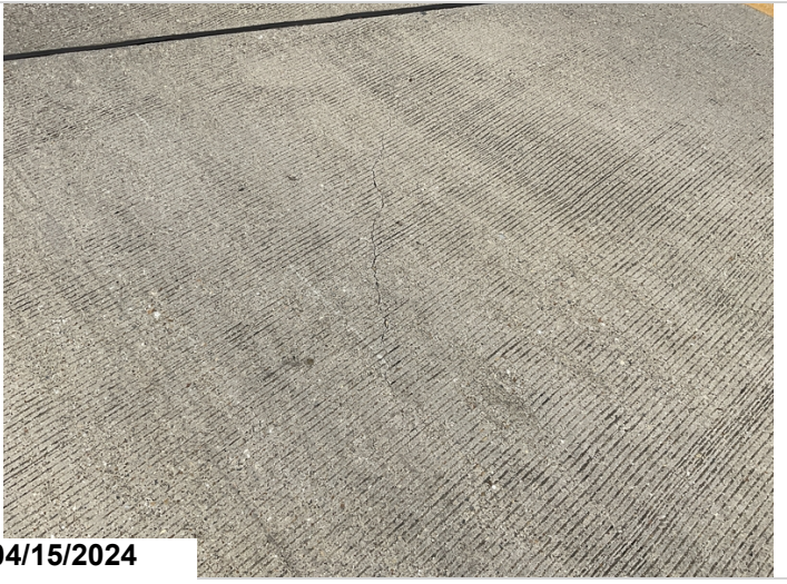
Span 3, Right side, Deck cracking, CS2.
