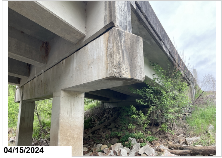
Bent 2, Looking back, Spalling to left side of cap, CS2
