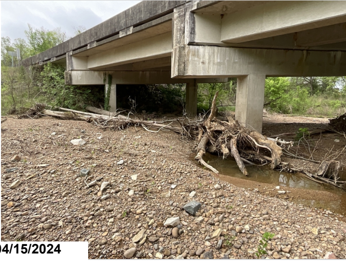
Log jam is located on the upstream side of intermediate bents 2 & 3.
