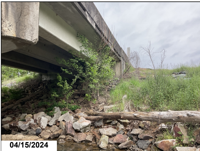
Beginning of bridge, Left side, Trees and vegetation growing over bridge railing.
