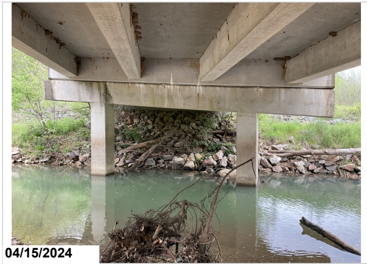
Cracking with efflorescence to concrete diaphragm at all bents
