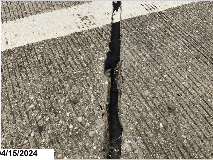
Bent 3, Right side, Loss of seal adhesion, CS2
