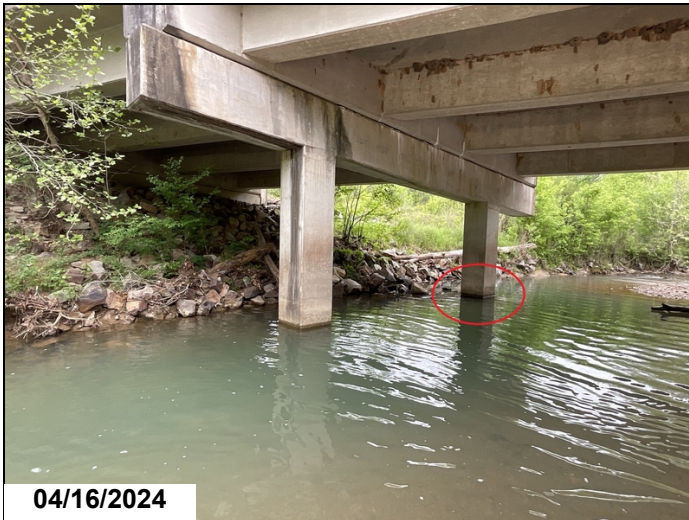
Scour area around bent 3, column 1.
