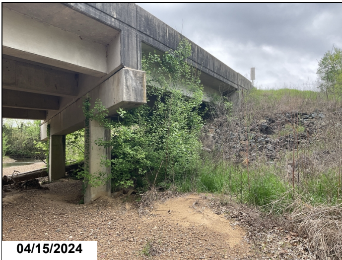
End of bridge, Right side, Trees and vegetation growing over bridge railing.
