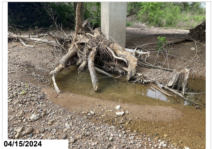
Bent 3, Column 1 scour from log jam.
