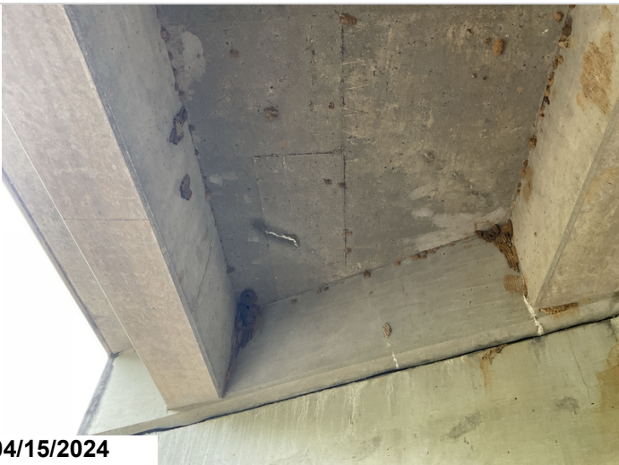
Span 2, Bay 1, cracking with efflorescence to undersurface, CS2.
